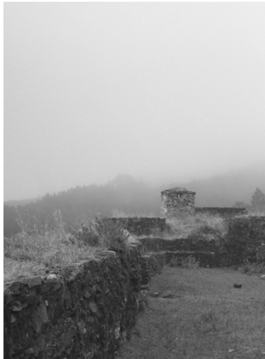
c.1948. Parapeto sur, cara interior
